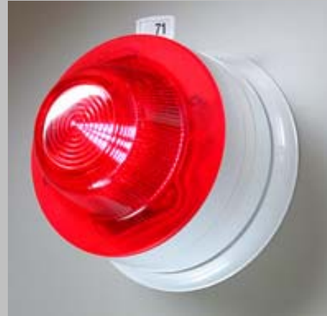
Loop-powered beacon clipped into the an integrated base sounder
